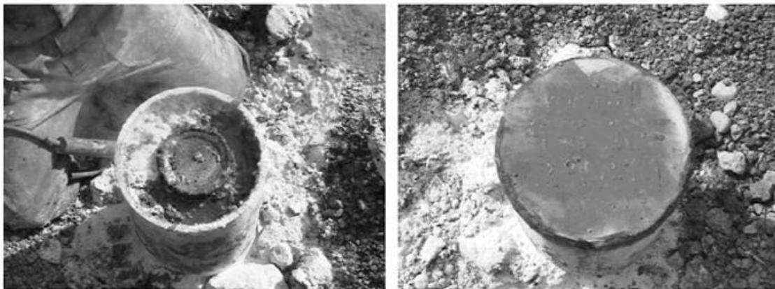
Figure 6: Illustration of wellbore cut and cap on production casing and surface casing.
