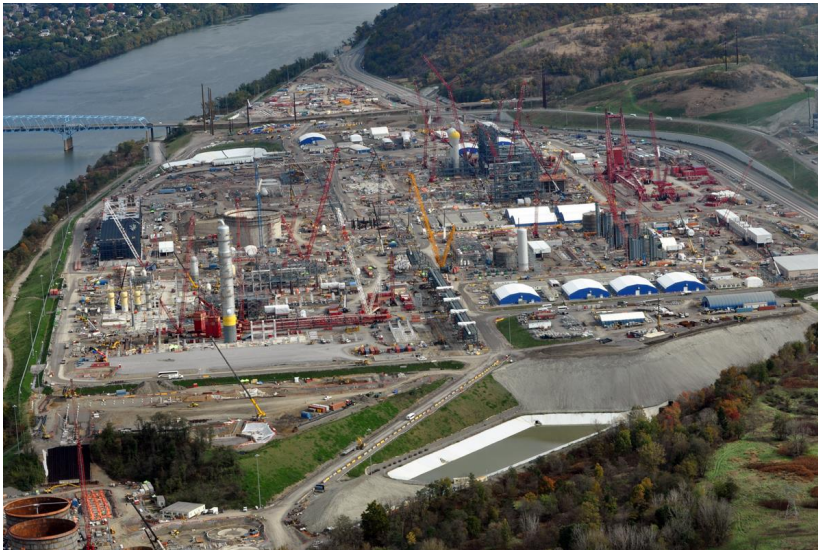
Beaver County Cracker Plant as of September 2018 Courtesy Marcellus Air
